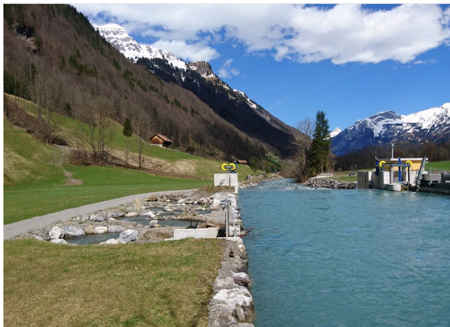
Skat Consulting supports the "Swiss Small Hydro" association. The photo shows an excellent example of an environmentally sound hydropower plant (fish pass on the left).
